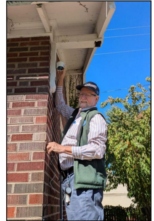
Gary Zuckett, WV CAG Co-Director , installs a PurpleAir monitor at the CAG office in Charleston, WV.
